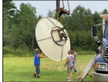
new, more stable pedestals are immune to the frost heave and new cable and hardware were also added to the project to ensure the highest possible signal quality.
